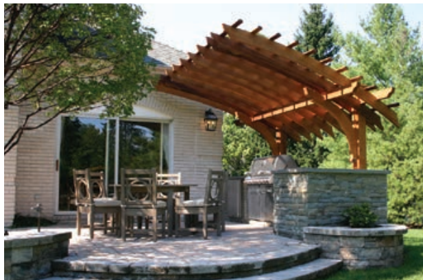
Unique cantilevered kitchen pergola which eliminates posts in the sitting and traffic areas
