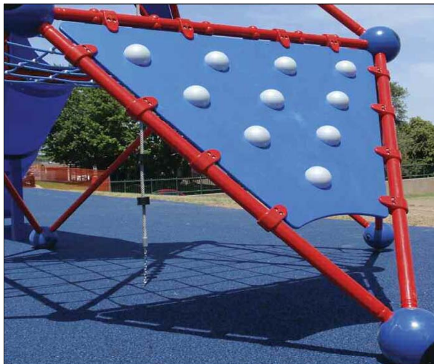
Check individual components for excessive wear, deterioration and potential hazards.
