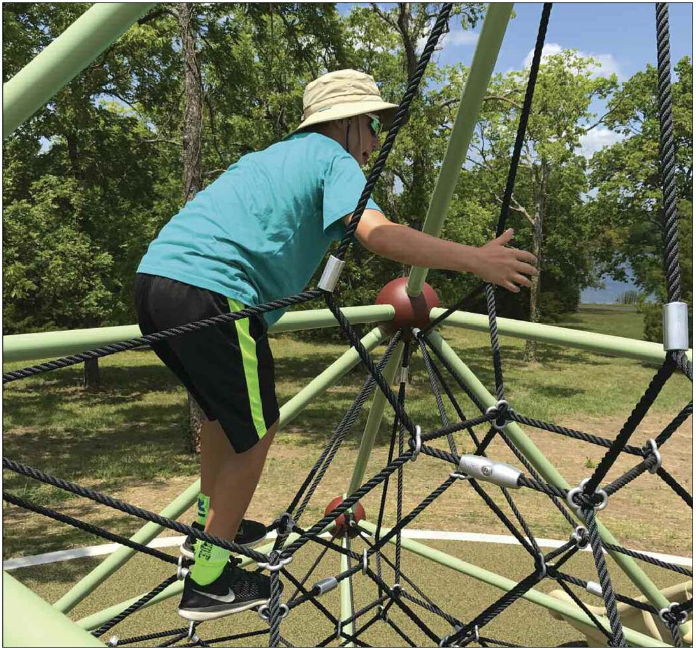
The ropes on rope play equipment will last longer if tensioning is maintained.
